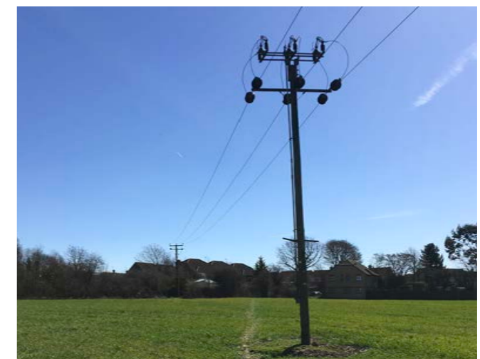
Overhead power lines
