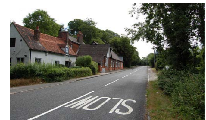
Looking east along Vicarage Lane West, with church and associated buildings on the left (view 4)
