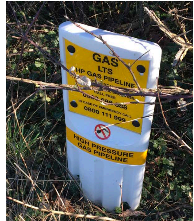
Gas pipeline marker
