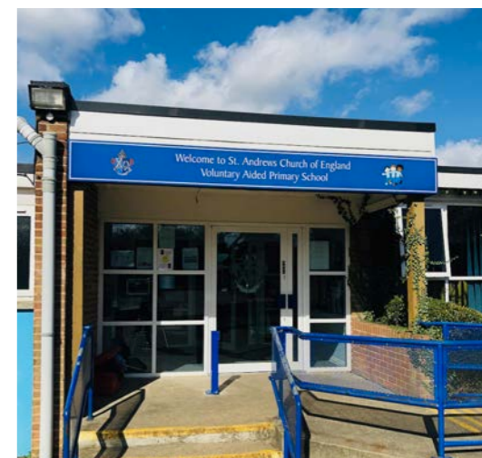
St Andrews primary school
